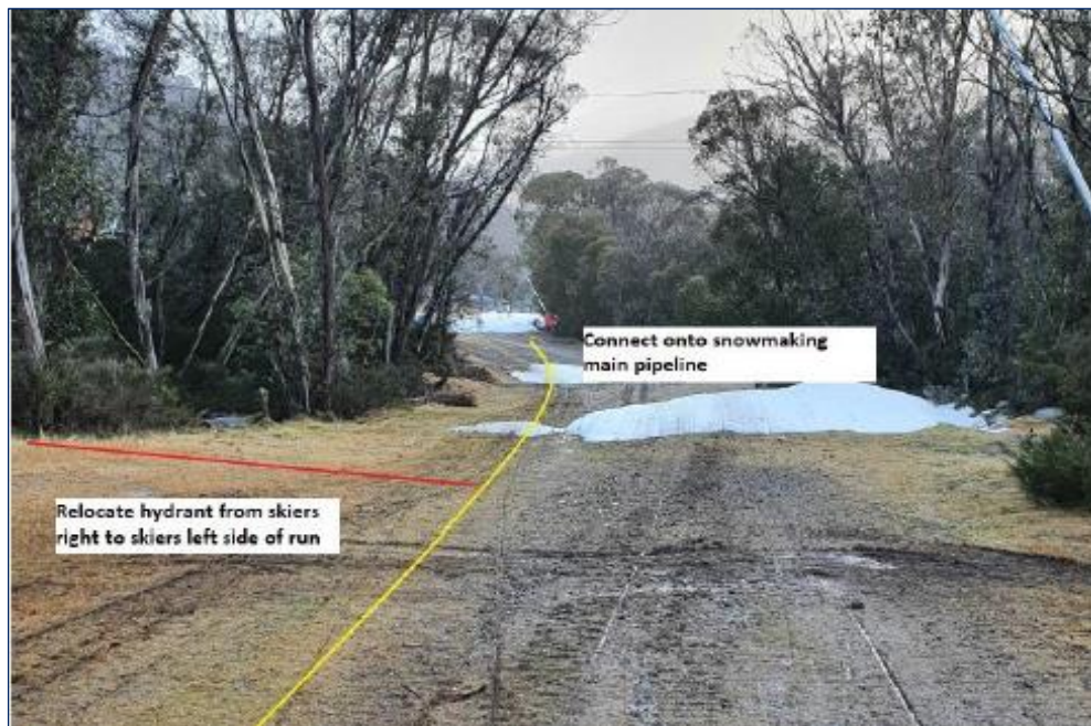
Figure 2 | Alignment of pipe and hydrants along Sundowner ski run (Source: Applicant's documentation)
