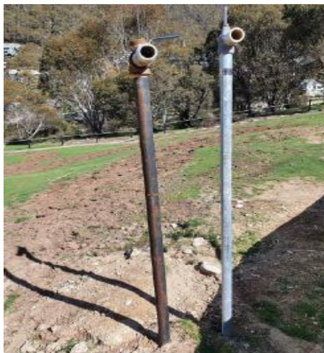
Figure 5 | Example of a manual hydrant installation (Source: Applicant's documentation)
